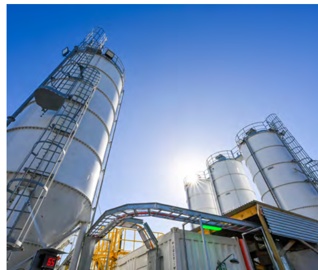
Image: The purpose-built water treatment plant at Rosehill that supplies all Tunnel Boring Machine operations with treated groundwater.
