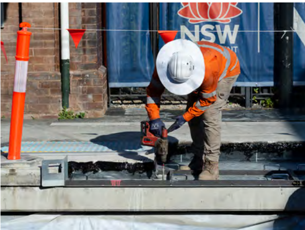
Image: Installation of mechanical gap filler at Hurlstone Park Station platform.
