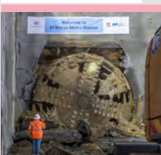
Image: TBM Catherine breakthrough at St Marys Station.
