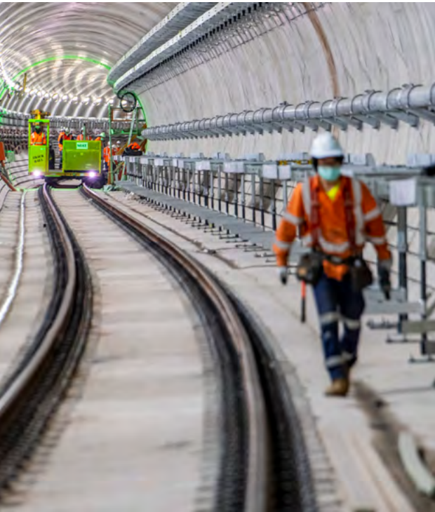
Image: A safety walkway is installed inside the Sydney Metro tunnels. The safety walkway will allow passengers and metro staff safe access to the cross passages and exits from the tunnel.
